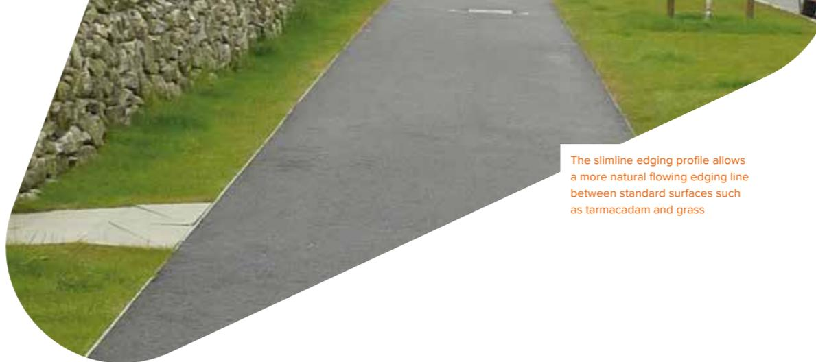
The slimline edging profile allows a more natural flowing edging line between standard surfaces such as tarmac and grass
