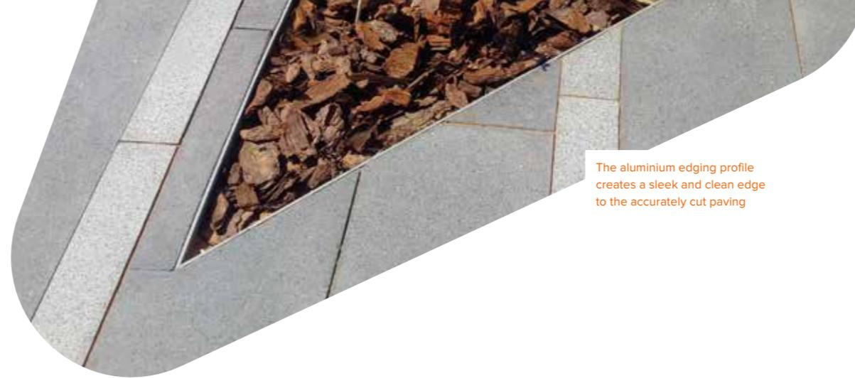
The aluminium edging profile creates a sleek and clean edge to the accurately cut paving
